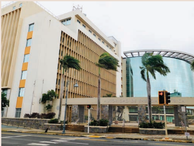
PREPA's headquarters, Santurce, San Juan, Puerto Rico.
