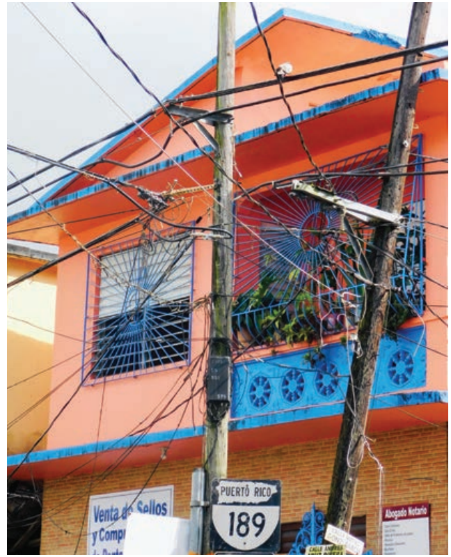
Current state of poles and wires part of the PREPA's distribution system. Gurabo, Puerto Rico.
